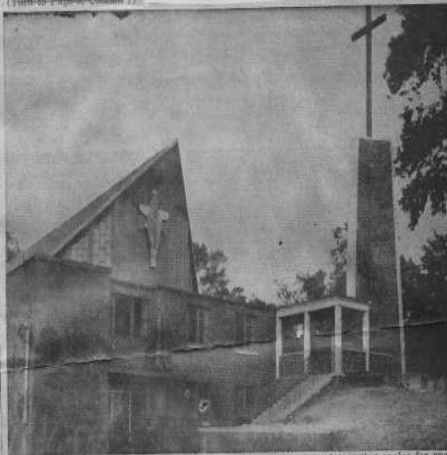
THE UNUSUAL LINES of Grace Lutheran Church provides many interesting angles for photographers, as indicated above. The new sanctuary will be formally dedicated tomorrow at 11 a. m. The church is located at Wayne Ave. and Thirteenth St. —(News-Virginian Photo)
