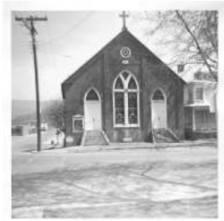
The church with the copper cross
